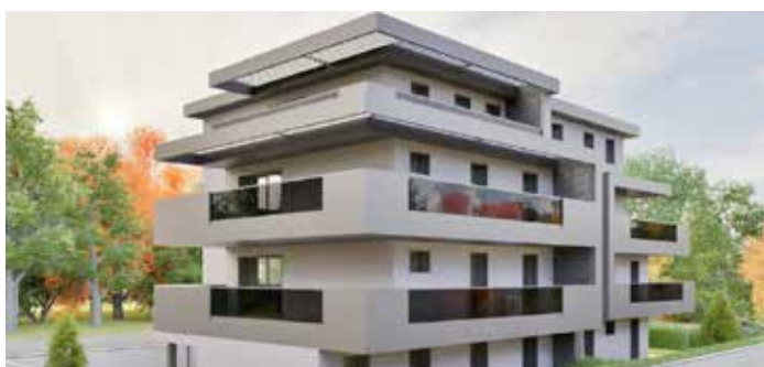
■ RESIDENCE IN VIA LATISANA
